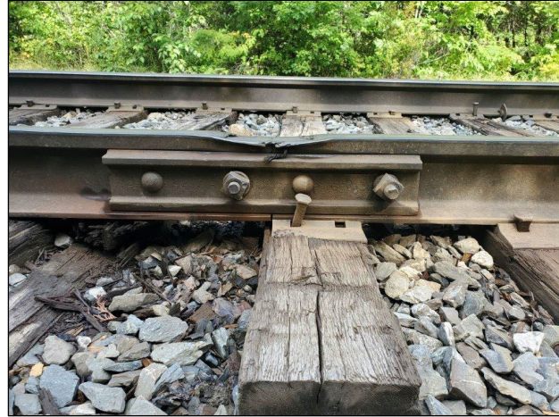
EMR track showing deterioration at a rail joint, compromising the strength of the track.
